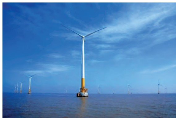
Figure 3-10 – The Shanghai Donghaidaqiao offshore wind farm (SGCC)
