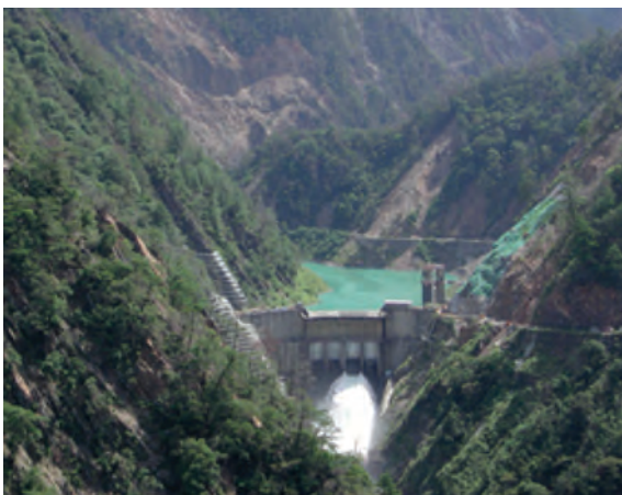
Figure 5-5 – A PHS plant in Taiwan [tem12]
