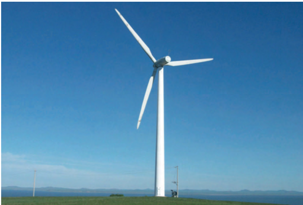
Figure 3-1 – A standard WTG with three blades and horizontal axis (SGCC)
