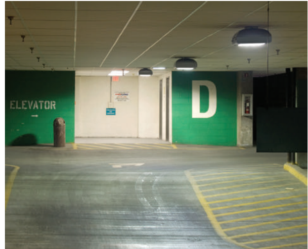
Figure 1 – Typical garage elevator lobby.
